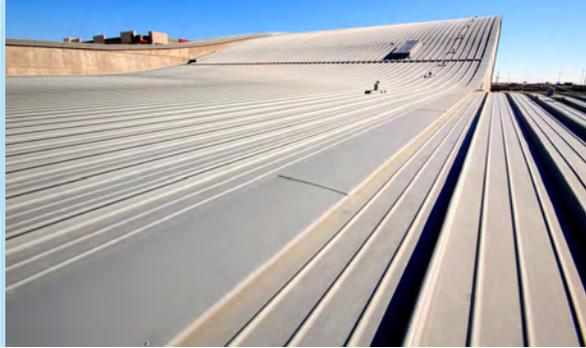
Left to right: A side view of the performance hall's unique multiwave, curved metal roof system; 10 layers of materials comprise the acoustic roof system.
