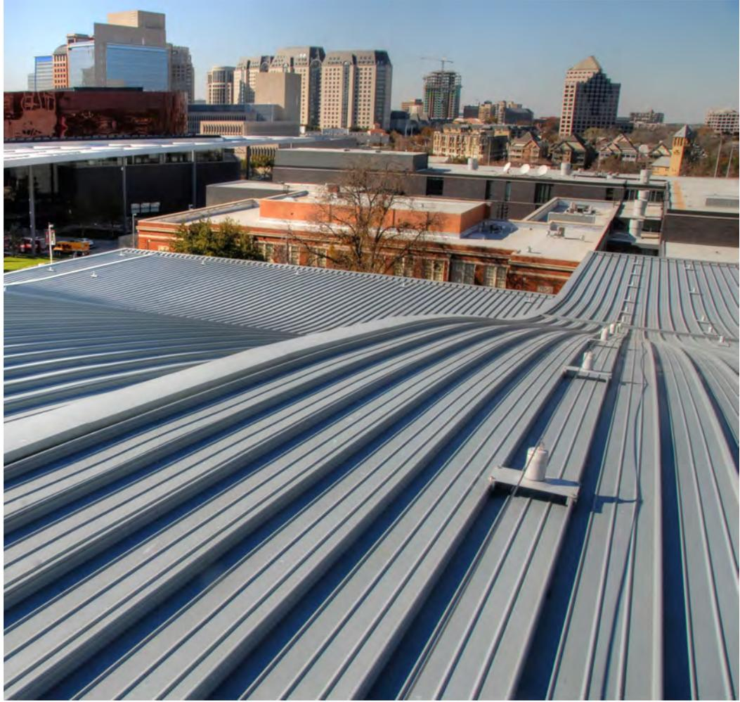
The Dallas City Performance Hall's roof system incorporated the longest Kalzip® single-length, roll-formed mechanically seamed AluPlusZinc panels in North America.
