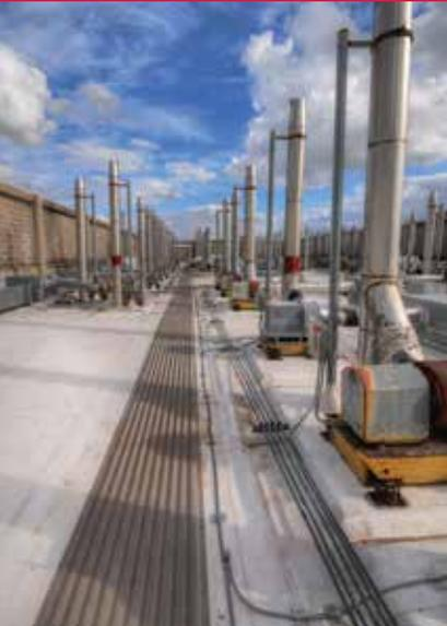
Top to bottom: 14,400 linear feet of electrical conduit was raised 1 inch before removing the old roof system and repositioned with new supports following the new roof system installation; 2,400 square feet of lightning protection was removed and reinstalled along with a new walkway for safety.
